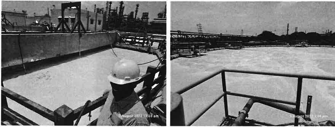
Whitish brown sludge in the aeration tank of ETP of MPL plant 1 (left) and plant 2 (right)
